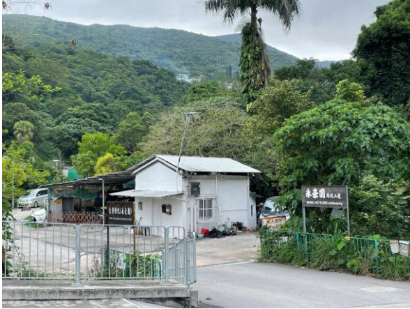
① Existing Access to the Application Site
